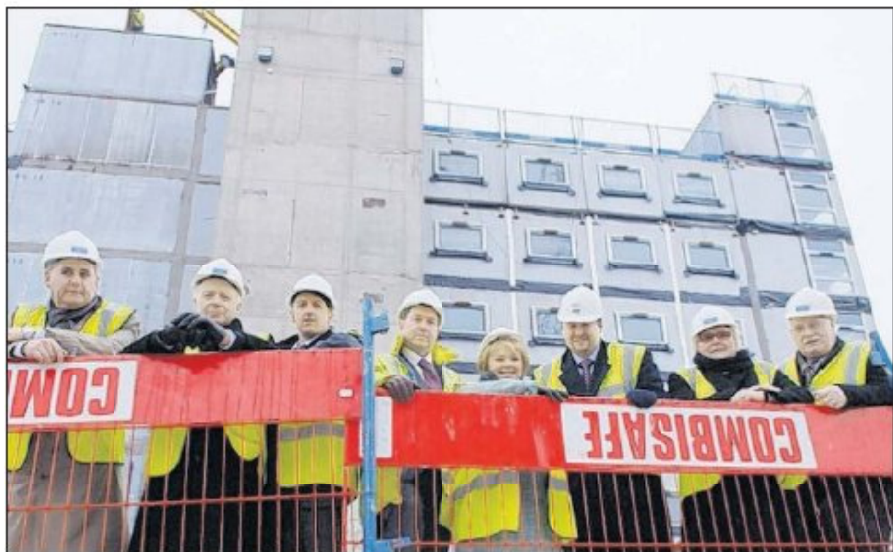
From left, Steve Boyes, Ian Oakes, David Salmons, Bob Crompton, Mayor Christine Mills, Will Evans, Paddy Bradley and Neville Patten at the Victoria Hall construction site
